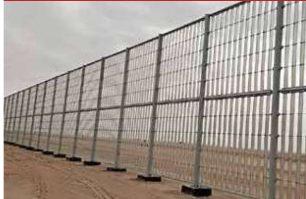
Mohammed Bin Rashid Al Maktoum Solar Park Phase-IV
